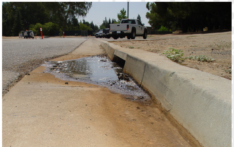
Storm drain at Woodward Park in Fresno.
